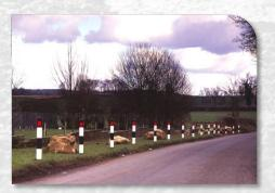
Traditional, rounded verge post made from hollow UV resistant polyethylene.
